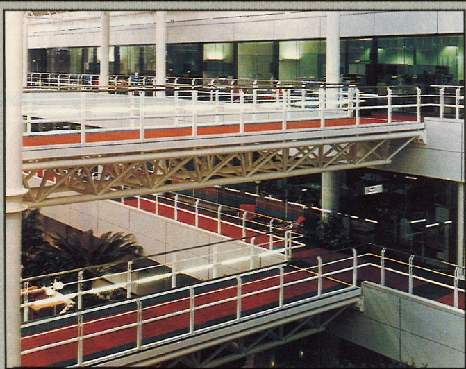
When architects, Percy Thomas Partnership designed the staircases and walkways for the Esso headquarters at Leatherhead, they needed a light fitting that could be totally integrated into the handrails, maintaining the style and following the contours of the stairs to illuminate the walkways at floor level.
